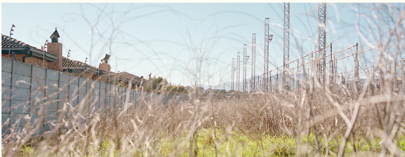
Dry shrubbery masks the substation that sits on the boundary line of the Burgundy suburbs and feeds the Teraco complex in Cape Town.
