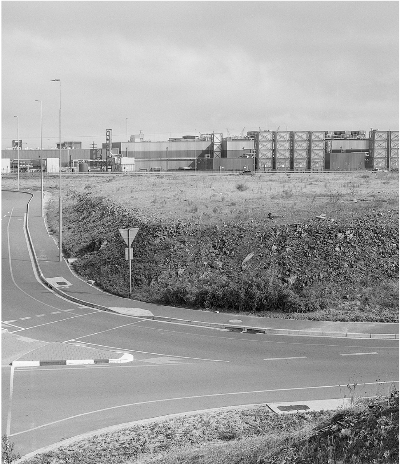
A view of the Atlantic Hills Data Centre with the newly built roads that service the area.
