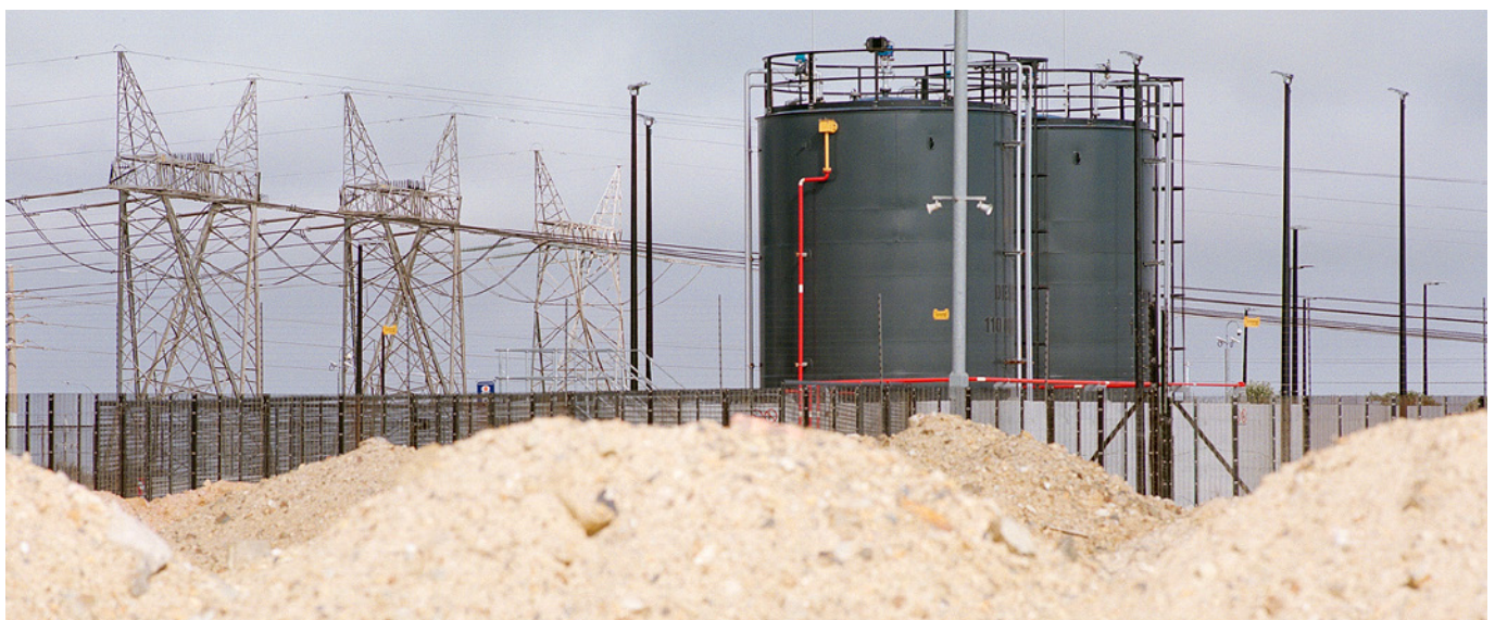
Sand mounds and building substrate for new construction next to the Atlantic Hills Data Centre.
